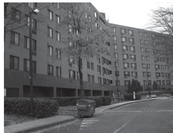
FOXWELL MEMORIAL APARTMENTS in West Baltimore
