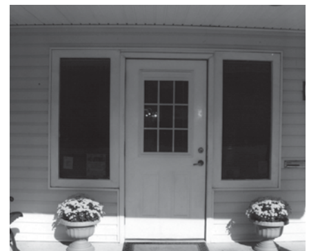
RIVERSIDE APARTMENTS in Columbia, SC
